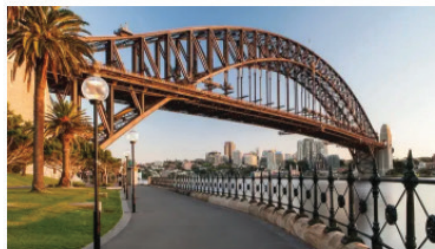
Sydney Harbour Bridge
